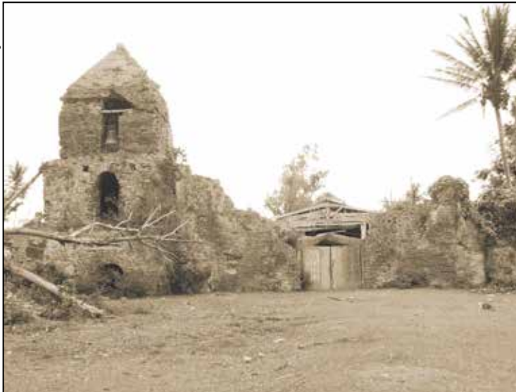
The broken façade faces west, and confronts the Cagayan River.
