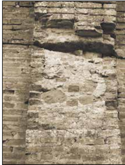
Buttress on the east end of the church where the brick cover has disintegrated, affording a view of the filling materials within.
