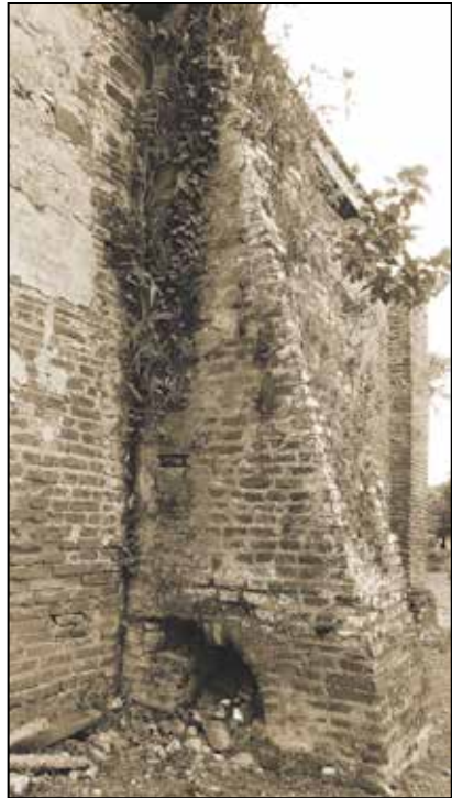
Unique open arch at the base of a buttress, just outside the apse.
