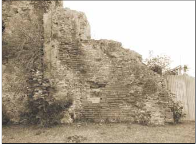
While the first two levels of the tower are of rough stone blocks, the rest of the church as well as the third level of the tower are of brick. A deep cleft between the tower and the nave shows that they were built at different times.
