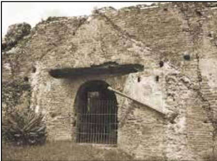
Entrance to the south side of the church; a substantial canopy must have been attached to the wall at one time.
