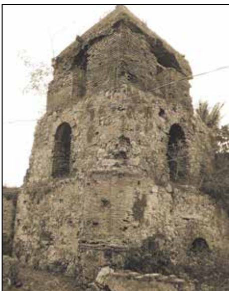
View of the tower from the northwest, showing the coupled columns of brick at the corner.
