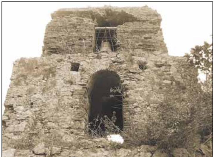
View of the second and third levels of the tower, of rough stone and brick respectively. The square holes may have held supports for an overhang over the second level window, or a balcony for the third level.
