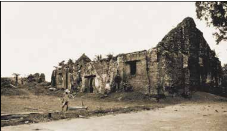
Buttress on the east end of the church where the brick cover has disintegrated, affording a view of the filling materials within.
