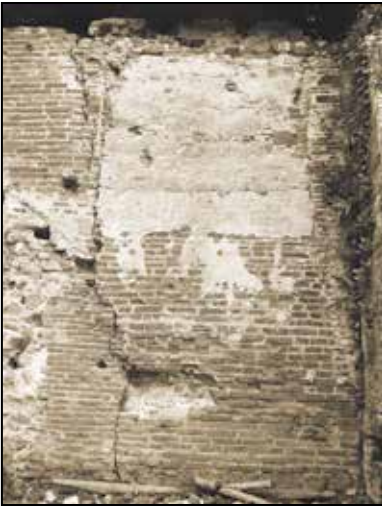
Portion of the south wall, corresponding to the apse. A window has been walled up.
