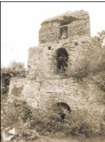
Closer view of the western side of the tower, which faces the river.
