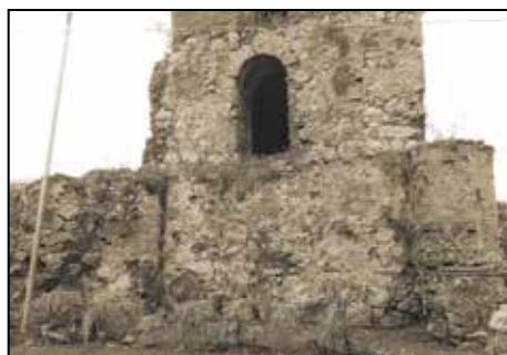
View of the northern face of the tower. Coupled columns of brick were constructed at the northwest corner (right) and northeast corner (left, in ruins).
