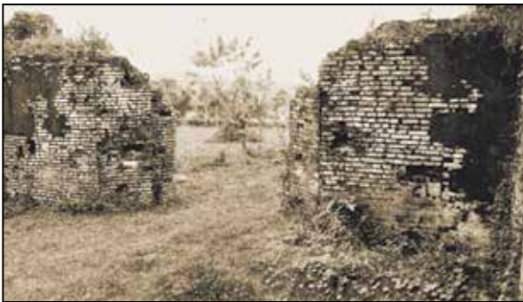
Main entrance, viewed from the nave.
