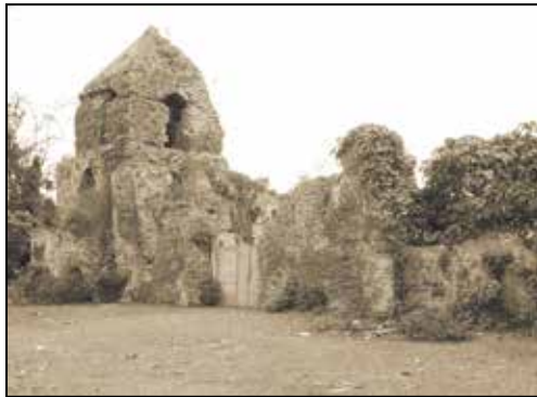
View of the church from the southwest.
