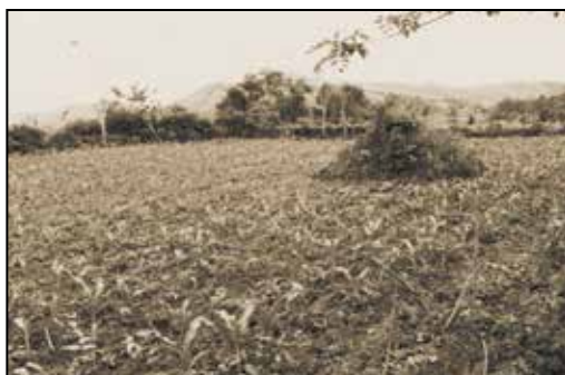
In the middle of the patio is the remnant of the pedestal for the atrial cross.
