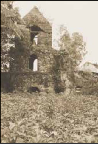
The bell tower is distinguished by its pyramidal masonry cupola, unique in the Cagayan Valley.
