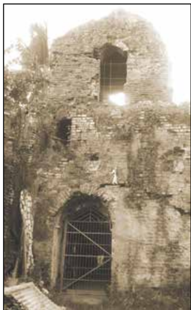
View of the tower from the nave, or the south side. Note the different heights of the entrance to the tower. The entrance from the nave is higher, while the original entrance of the tower itself is lower. The rectangular opening above this entrance led from the choir loft to the bell tower. The Dominican protomartyr San Francisco de Capillas would sleep on this choirloft.
