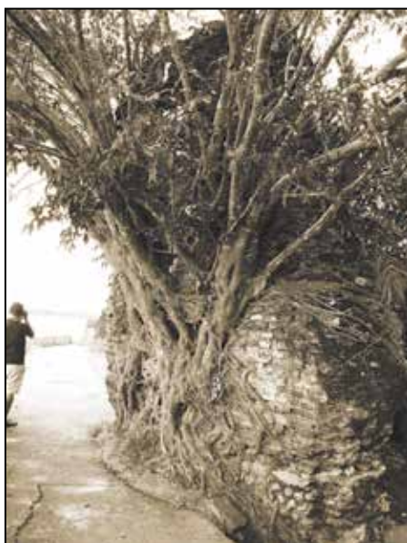
Ruins at the rear of the church. The balet roots engulf what seems to be a buttress.
