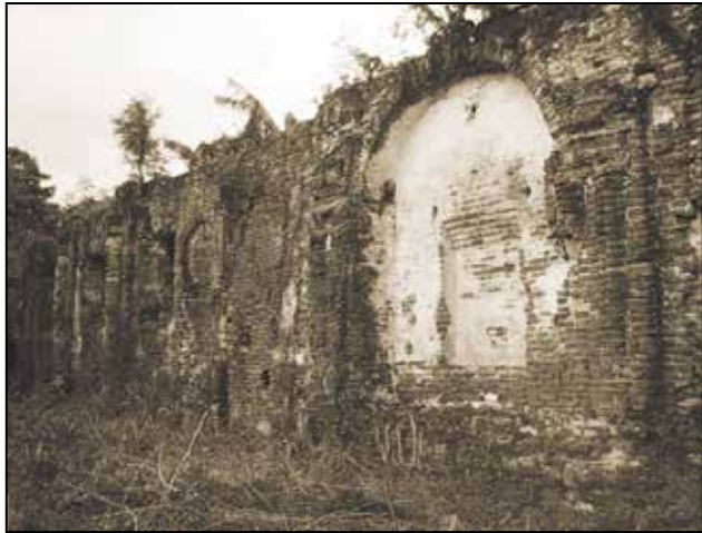
Another view of the inner face of the eastern wall.
