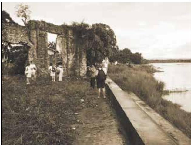
View of the end of the eastern wall, cut short by the embankment by the river.
