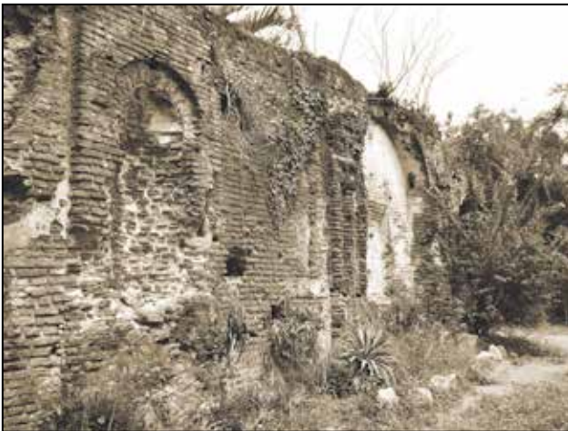
Closer view of a section of the eastern side.
