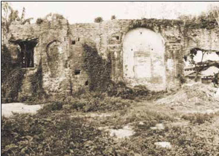
Frontal view of the same section, showing the site where the pulpit used to be, and a wall still with its palitada where a retablo probably stood.
