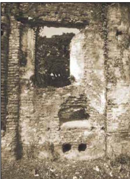
Wall to the right of the “entrance,” featuring a large window. The empty niche may have served as a tomb for bones. The two smaller holes may have held the ends of beams, which may have supported the floor boards for the main altar area.
