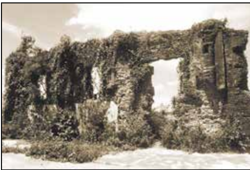
View of the inner face of the western wall.
