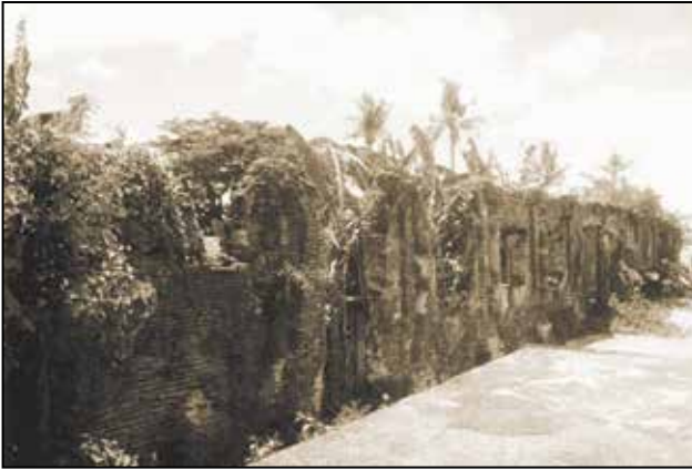
Interior wall of the eastern side of the nave.
