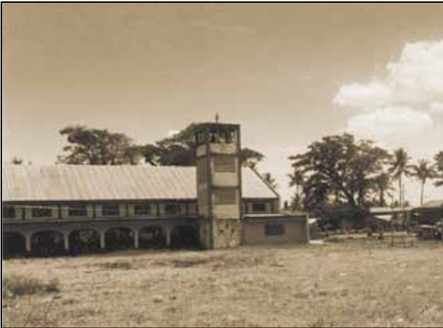
The new church was built perpendicularly to the ruins, away from the river.
