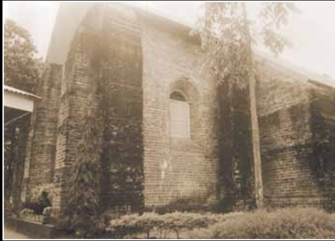
Apse (rear end) of the church.
