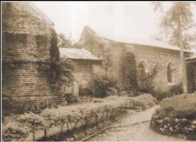
View showing the apse (left) linked by a passage (center) to a chapel (right).
