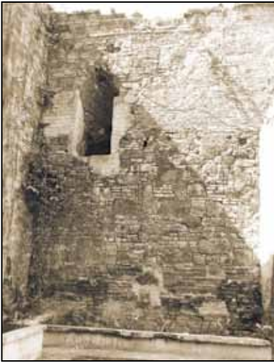
Left wall of the narthex, a vestibule between the façade and the main part of the nave. The narthex was separated from the longer part of the nave by the choir loft arch. The arched opening linked the choir loft to the stairway that led to the ground level.
