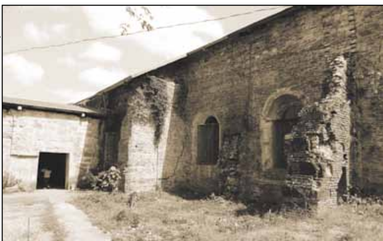
Exterior of a section of the left flank of the nave, corresponding to the left “transept.” The other side of the old convento may also be seen. The buttress left of center has an angled silhouette. The one to its right is unique in the church for the inclusion of cut stone in a basically brick support.
