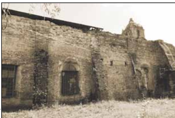
Exterior of a section of the left flank of the nave, corresponding to the left “transept.” The other side of the old convento may also be seen. The buttress left of center has an angled silhouette. The one to its right is unique in the church for the inclusion of cut stone in a basically brick support.
