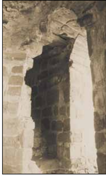
Passage from the third to the fourth floor, adhering to the walls.
