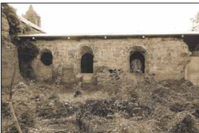
View of the same side of the convento, this time with the stones cleaned. Note that the lower portions are of brick; it seems that when the brick walls crumbled they were rebuilt with cut stone.
