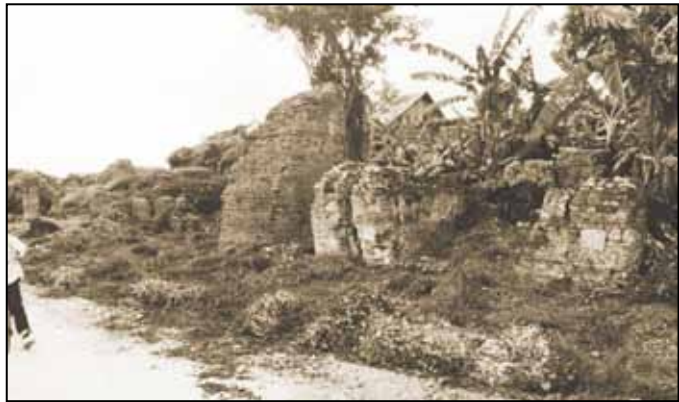
Ruins of a large brick convento nearer the façade of the church. A brick buttress can be observed, as well as a masonry enclosure.
