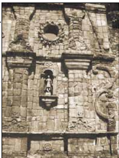
Right section of the façade.
