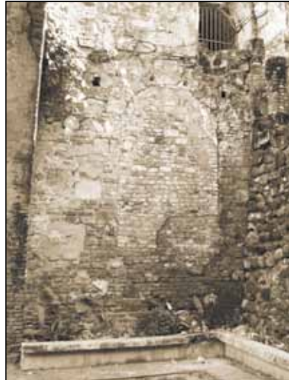
One can discern a door or window that has been walled up, as one inspects the right wall.
