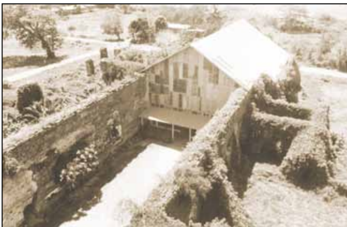
View of the nave, apse, and right chapel from the bell tower.
