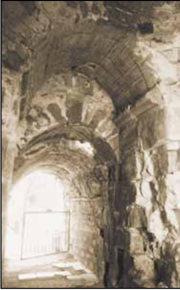
Passage from the second level of the tower to the church. Note the different types of stone and brick construction of the walls, indicating different times of construction.
