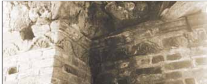
Passage from the second level of the tower to the church. Note the different types of stone and brick construction of the walls, indicating different times of construction.
