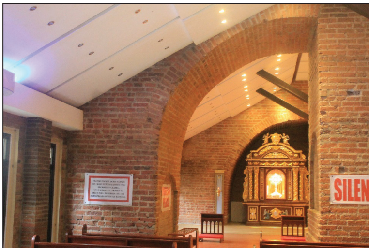
Figure 21. Northern flying buttresses (showing the intrados) now part of Tuguegarao Cathedral's Adoration Chapel. Photo: M. T. Tabao, 2022.
