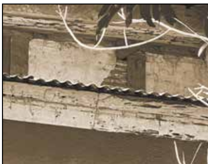
Fig. 14. Tabique pampango on upper section of the convento, Matalom, Leyte.
