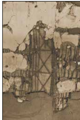
Fig. 29. Close-up of the boards wound with rope, and with clumps of lime plaster.
