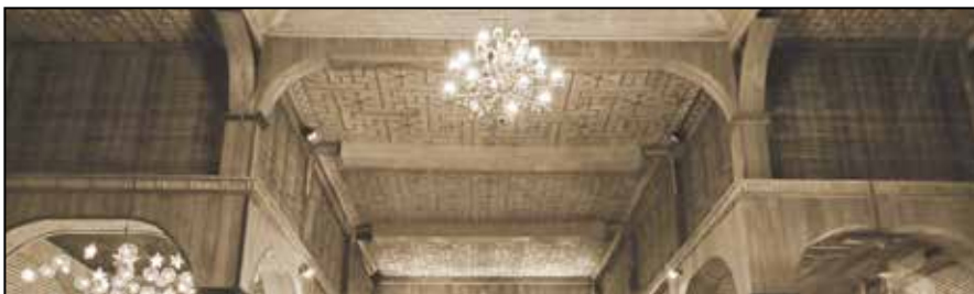
Fig. 34. Most of the wattle was installed by Christmas, 2023.
