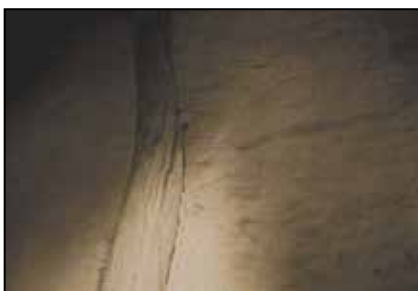
Fig. 9. View of a wall in the convento of Badian, Cebu. The bamboo wattle can be discerned under the daub.
