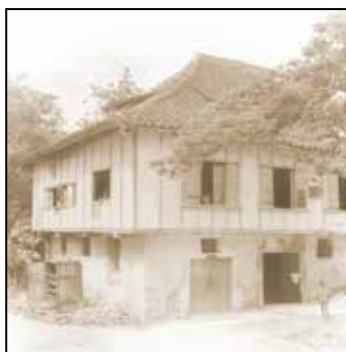
Fig. 23. Convento of Oslob, Cebu. Most of the plaster is still intact, concealing the board-type of tabique pampango .
