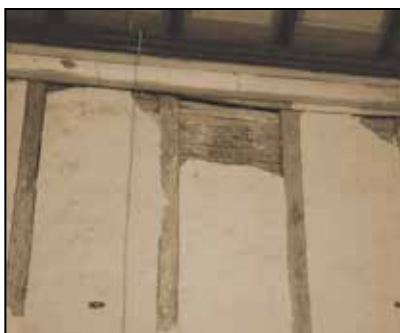
Fig. 22. Board-type of tabique pampango in convento, Dalaguete, Cebu.
