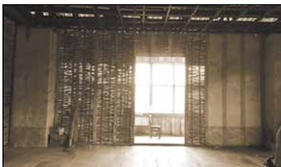
Fig. 4. View of wall, where the lime plaster has been stripped off sections of the wattle. The intact sections are painted white and indigo.
