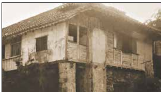
Fig. 21. Board-type of tabique pampango at one of the convento, Boljoon, Cebu. Sections of the plaster are still extant.
