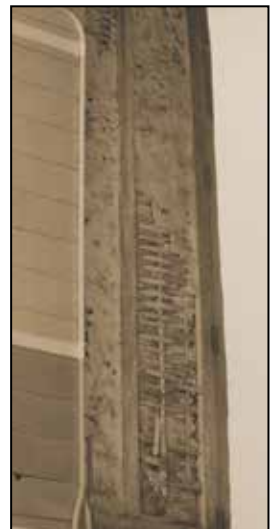
Fig. 10. Close view of the tabique pampango linking the church with the convento, Nueva Caceres, Cebu.
