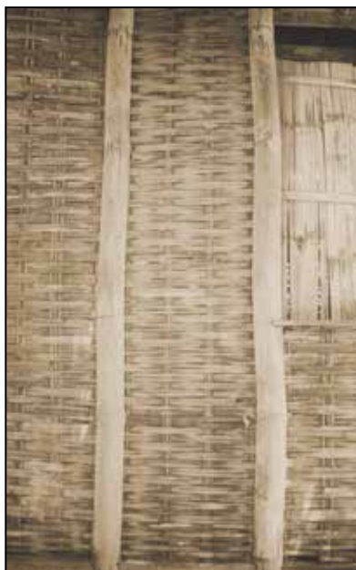
Fig. 3. A wattle of bamboo, seen in a house near the parish church, Oslob, Cebu.
