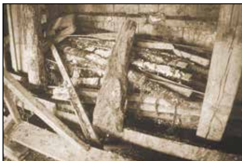
Figs. 24, 25. Remains of wood boards from discarded tabique pampango wall in the apse of the church of Jabonga, Agusan del Norte, with remnants of cabo negro and lime plaster.
