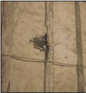
Fig. 7. Tabique pampango partition wall in convento, Baclayon, Bohol.
