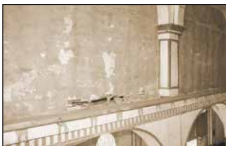
Figs. 16, 17. Tabique pampango in the upper section of the nave of the church, Jasaan, Misamis Oriental.
