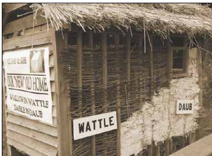
Fig. 1. Basic technique of wattle and daub.
