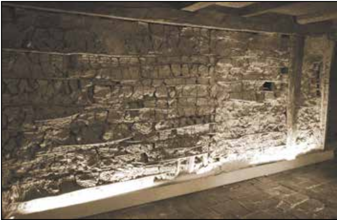
Fig. 2. An inner wall of pau-a-pique in the Monastery of the Immaculate Conception of Light, built in 1774. São Paulo, Brazil.
