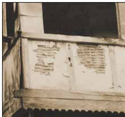
Fig. 31. Bamboo wattle showing through the plaster of the arcaded gallery.
