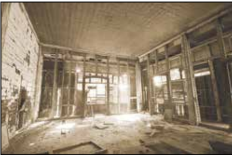
Fig. 26. Central hall in the convento.
