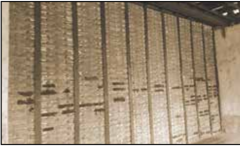
Fig. 5. Back view of unplastered wall.
