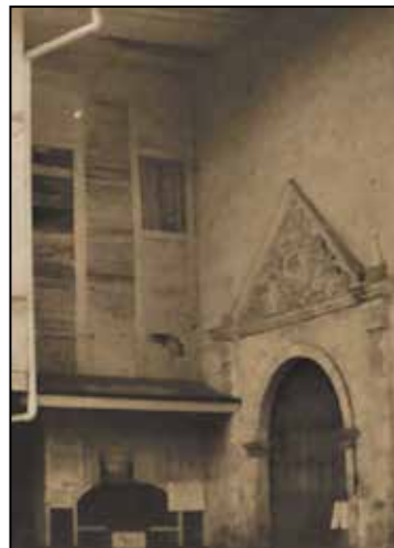
Fig. 20. Board-type of tabique pampango in junction between convento and church, Argao, Cebu.
