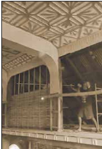
Fig. 33. Re-installation of tabique pampango in Jasaan.
