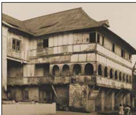
Fig. 30. General view of the convento. The bamboo tabique pampango is used for the arcaded gallery fronting the road. The board-type tabique pampango is used for the sides of the same gallery and the junction with the rear of the church.
