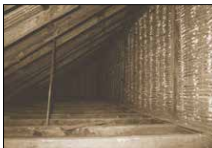
Figs. 16, 17. Tabique pampango in the upper section of the nave of the church, Jasaan, Misamis Oriental.
