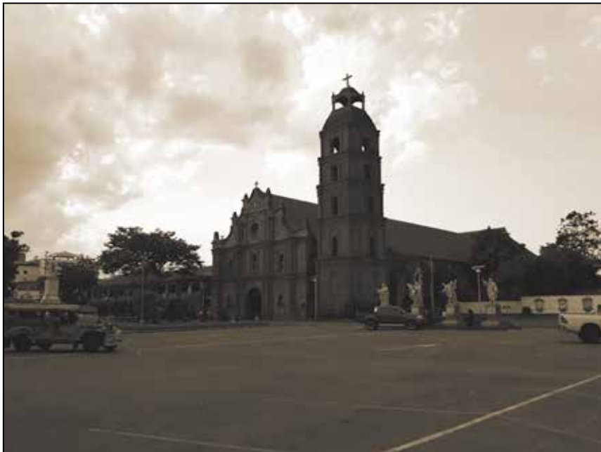
The façade and belfry of the Saint Peter’s Cathedral, Pastoral Center (formerly the convento ) and the paved patio at sunset.
