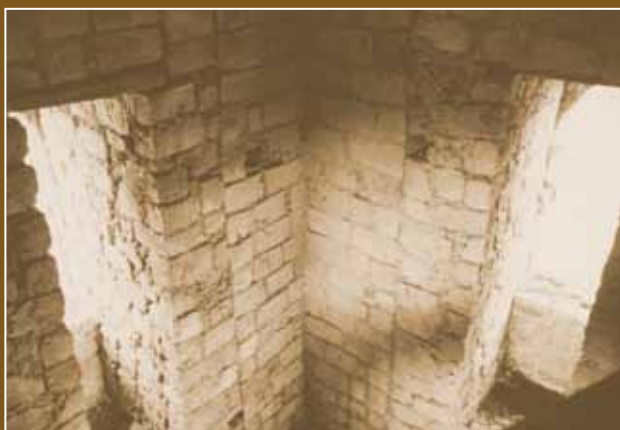
As seen from the stonework inside the bell tower, there seem to have been at least two stages in its construction.
