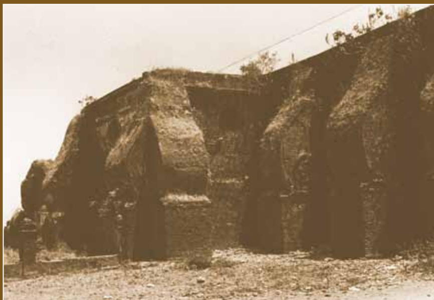
The enormous buttresses of Paoay are uniquely formed along the lines of volutes.
