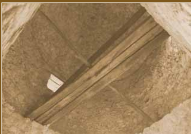
Inner view of the dome of the tower
