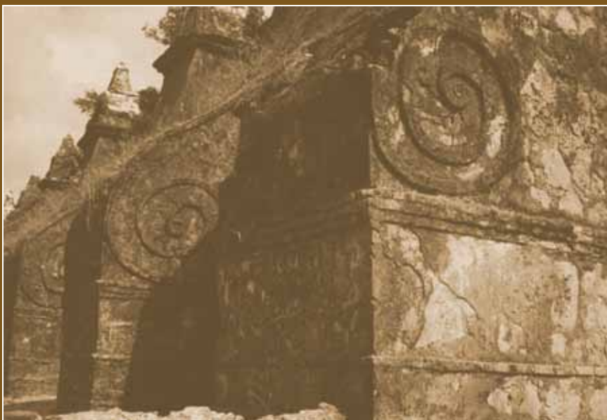
The enormous buttresses of Paoay are uniquely formed along the lines of volutes.
