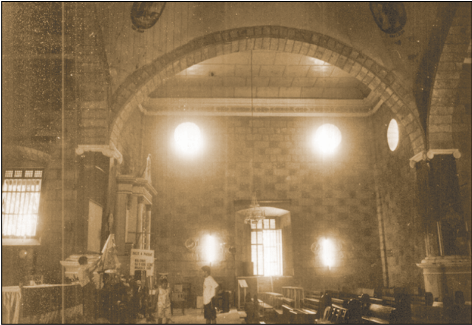
The checkerboard pattern of the bricks and stones can be clearly seen in this view of the right transept
