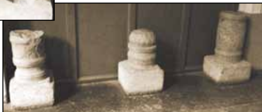
Remnants of stone balusters that bordered the first flight of steps of the main stairway. Now mounted in front of the UST Museum, Main Building, Sampaloc, Manila.
