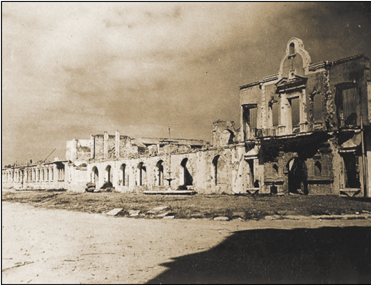
A victim of the Liberation of Manila from the Japanese in 1945, the old building was a total ruin. The Benavides monument was transferred to the Sampaloc campus and inaugurated there on November 13, 1946.
