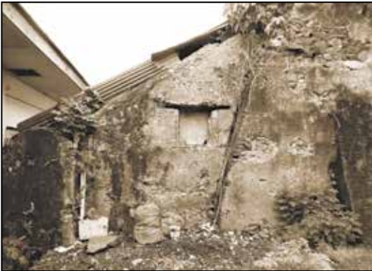
Right side of the apse, showing the junction with the sacristy.
