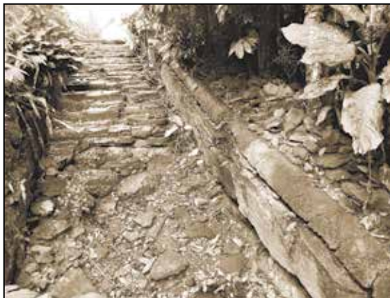
View of the brick stairway opposite the convento leading to the river, built by Father Santiago Capdevila, O.P.
