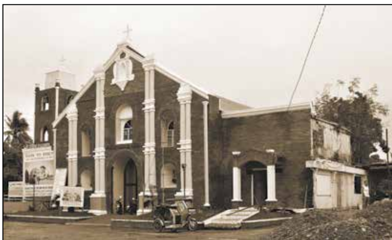
Church and convento, with recent brick tile overlay.
