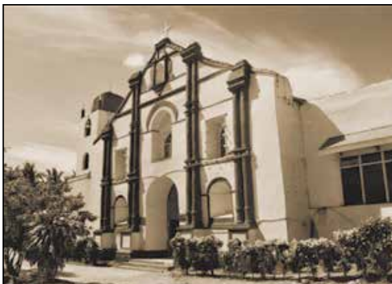
Church façade, with concrete finish.
