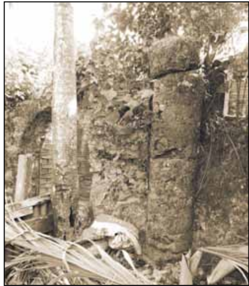
A round column flanking the inner side of the small door.
