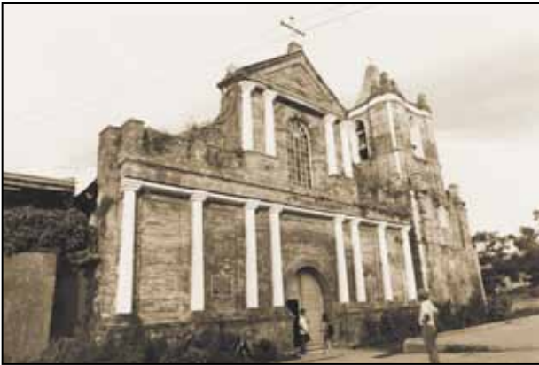
Church and tower seen from the northwest.
