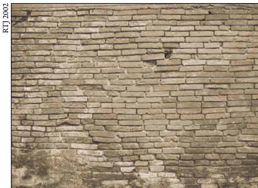
Section of brickwork at the apse.
