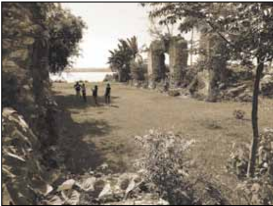
View of the nave looking from the apse towards the empty façade, with a view of the Cagayan River beyond.
