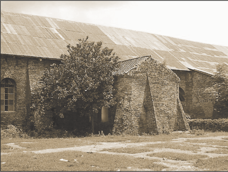
The chapel extension has retained its tile roofing.
