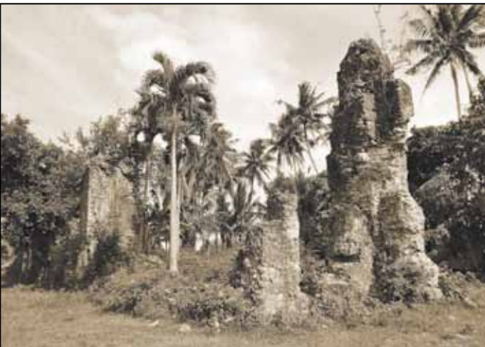
South-western corner of the collapsed façade, with the tall remnants of a possible bell tower to the right.
