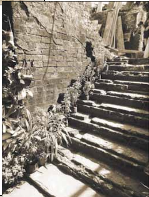
Stairway to the second floor, now demolished.
