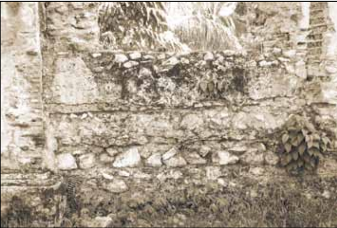
Detail of the wall, showing the alternating brick and stone courses.
