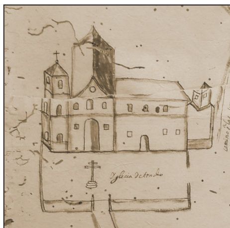
Figure 10. Convent and church of the Augustinians in the Chinese quarter (parian) of Tondo. The convent of two floors appears at the right side of the church.
