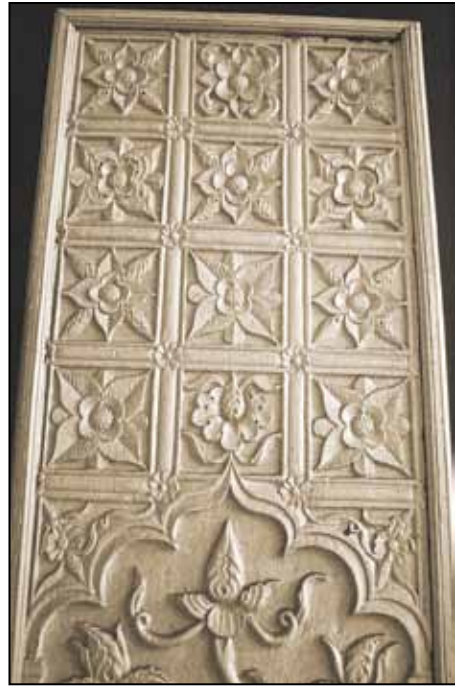
Section of a door leading from the vestibule to the convento in the parish church of Santiago Apostol, Bolinao, Pangasinan. 17 th -18 th centuries.
