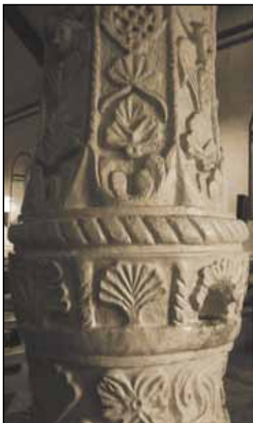
Lower section of a pillar supporting the choirloft in the parish church of San Vicente Ferrer, Dupax del Sur, Nueva Vizcaya. 1780s.
