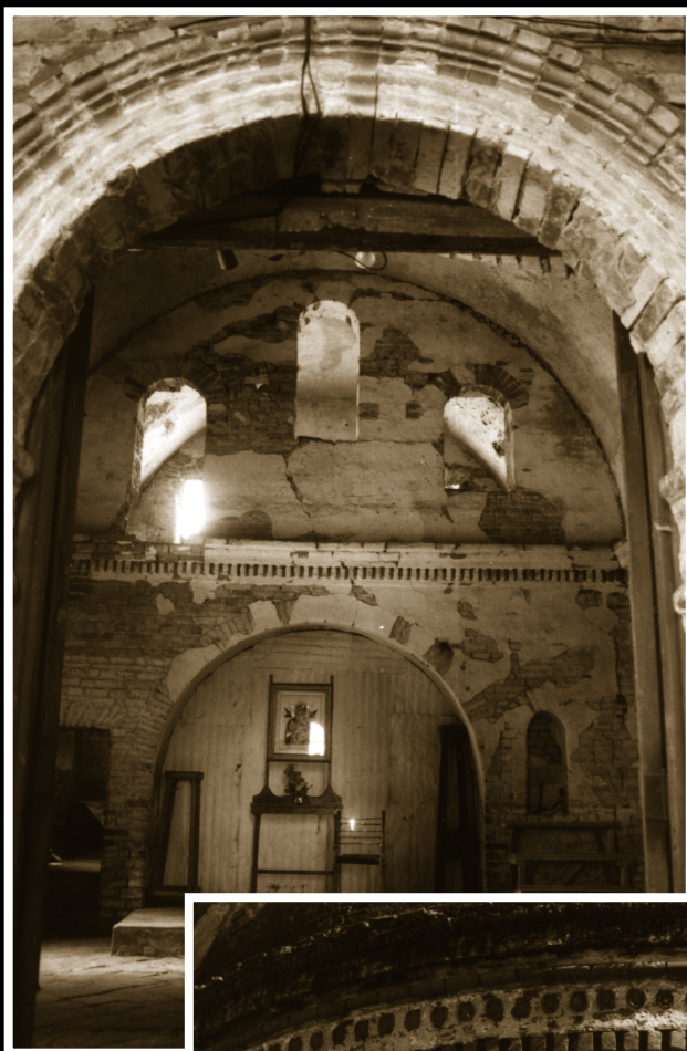
Interior of the sacristy, with its unusual "trinity" of windows. There is room at the back for storage.
