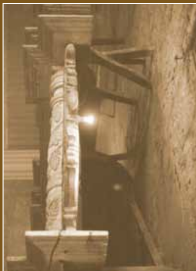
View behind the Santo Entierro retablo, showing its attachment to the wall.
