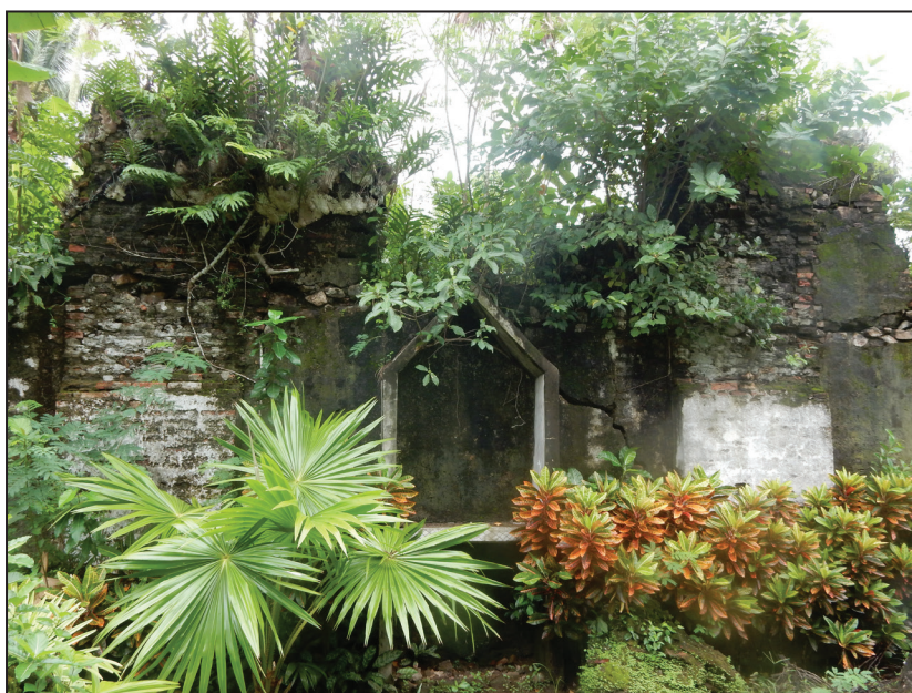
Fig. 15. Closer view of the nave, showing robust brick pilasters supporting the walls which still retain their palitada (lime plaster). RTJ 2017
