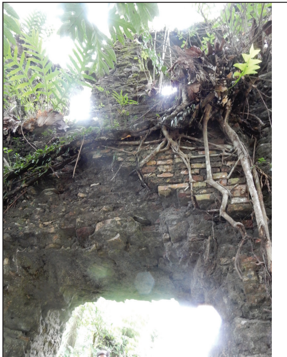
Fig. 11. Upper arch of the base of the tower. Note the brick cladding over the rubblework. RTJ 2017
