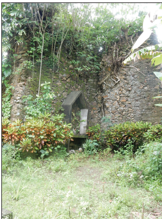
Fig. 14. Closer view of the apse, showing rubblework walls. RTJ 2017
