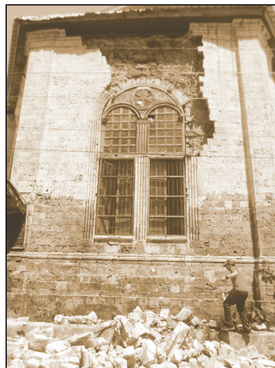
View of the choirloft, showing the early 20th century addition (white walls) over the darkened 19th century coralstone walls. The heaviness of the later concrete may have added to the destruction of the facade.
