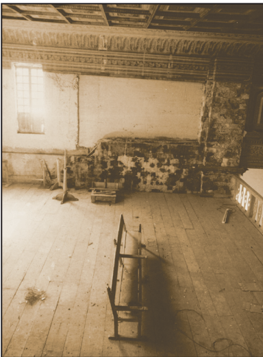
View of the choirloft, showing the early 20th century addition (white walls) over the darkened 19th century coralstone walls. The heaviness of the later concrete may have added to the destruction of the facade.
