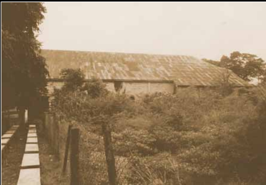
Fig. 9. Southern flank of the nave, with the extension of the apse introduced in middle of the 19th century.
