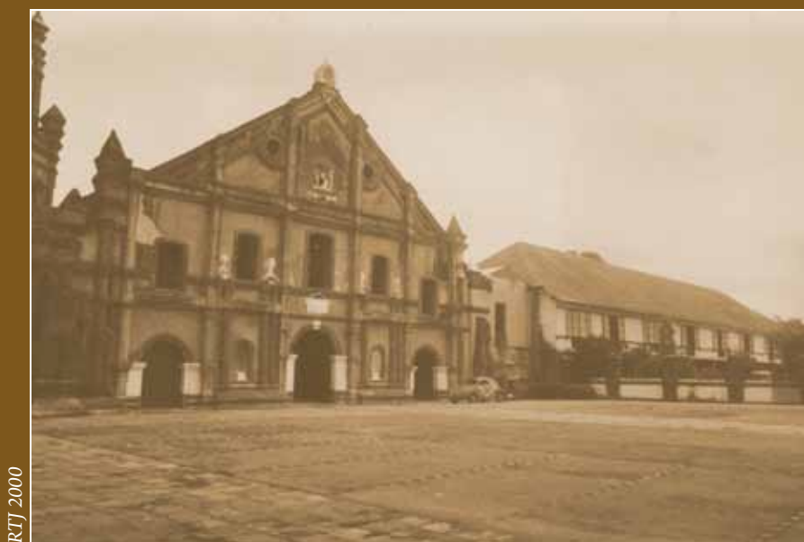
Fig. 5. Façade and convento , with the expansive church plaza.
