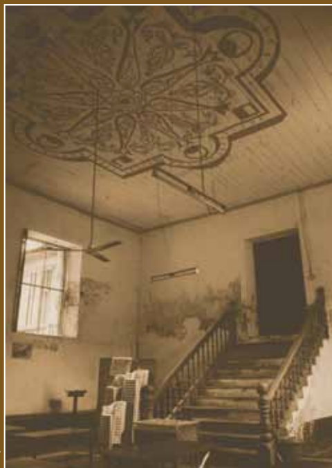
Fig. 34. Stairway leading to the upper level of the convento . The black and white design on the ceiling is similar to others found in northwestern Luzon buildings.
