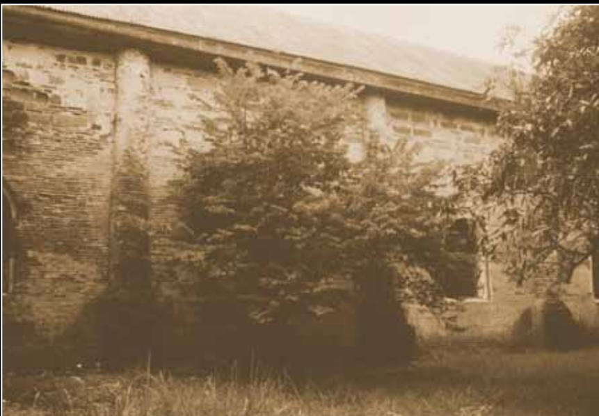
Fig. 10. Section of the southern flank, showing the addition of cut stone blocks over the brickwork. The column-like buttresses with stepped bases are similar to those in other Pangasinan churches.
