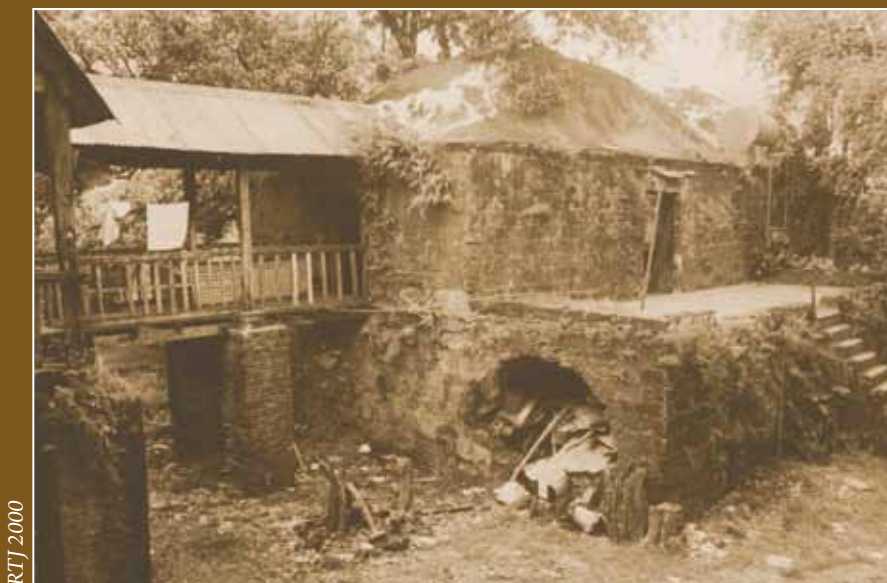
Fig. 37. The kitchen complex, built separately from the convento . The ground level is composed an aljibe (cistern) and arched storage tunnel for firewood and timber. A covered bridge on brick columns links it to the convento , while stone steps lead to the garden. The roof resembles a huge inverted vat.
