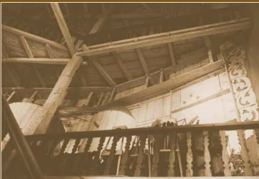
Fig. 17. Rear view of the central retablo . The backs of two niches may be seen, as well as the openwork flange to the right.
