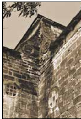
Fig. 9. Scroll buttresses supporting the quadrangular dome
