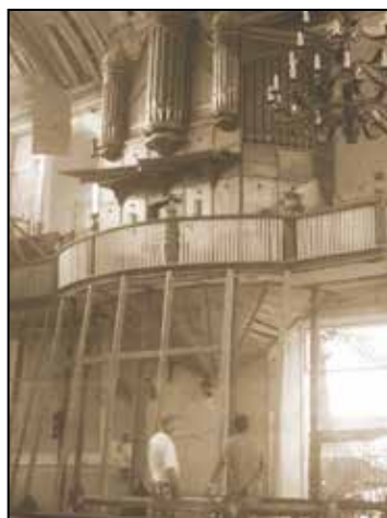
Fig. 19 The organ of Loboc was leaning forward after the earthquake. To prevent it from collapsing, bamboos were placed beneath. (Picture taken before it was dismantled in 2014)
