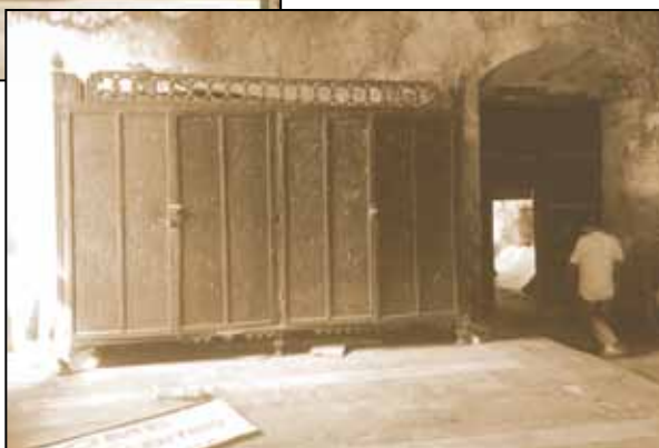
Rear of the convento , showing walls made of tabique pampango . This building was constructed under the direction of Fr. Manuel Carasusan, O.A.R., parish priest from 1842-1855, and again, from 1858-1864.
