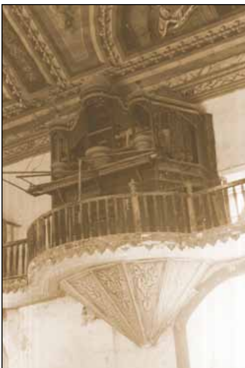
Pipe organ in the organ loft next to the choir, before its restoration.
