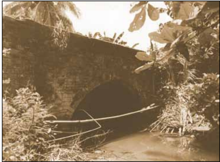
Bridge on the road linking Dimiao to Valencia.
