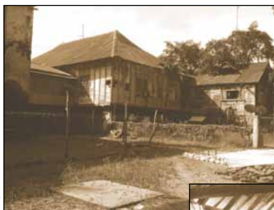
Rear of the convento , showing walls made of tabique pampango . This building was constructed under the direction of Fr. Manuel Carasusan, O.A.R., parish priest from 1842-1855, and again, from 1858-1864.
