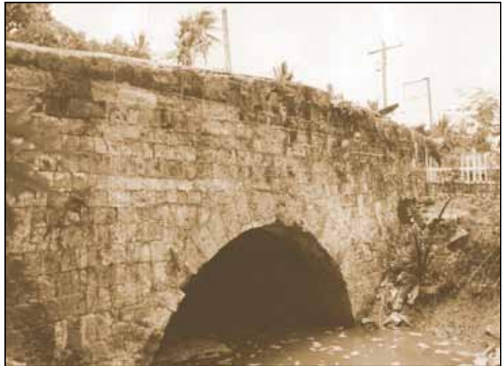
Another bridge on the same road, viewn from the side.
