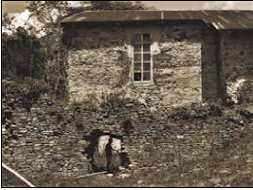
The outer and inner apses of the church at Malaueg (now Rizal), of rubblework and brick.
