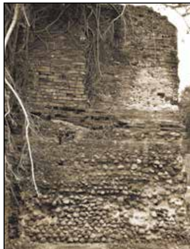
Section of a wall of the ruined convento, showing a lower level of rubblework and an upper level of brick.
