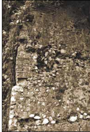
Section of a wall of the church of Tabang, Cagayan, of rubblework and brick.
