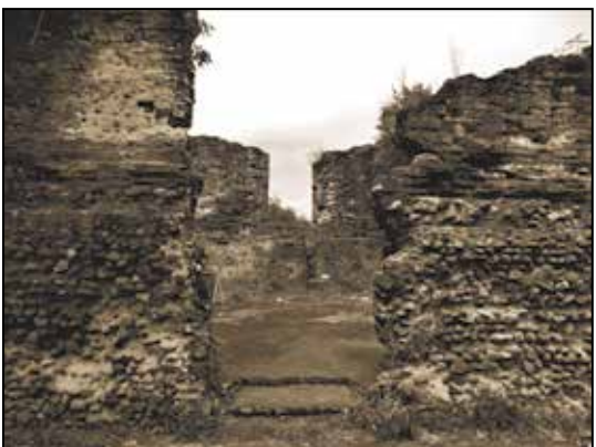
Another section of the convento. In the foreground is a wall with a passage way, of rubblework and brick. In the background is a wall completely of brick.
