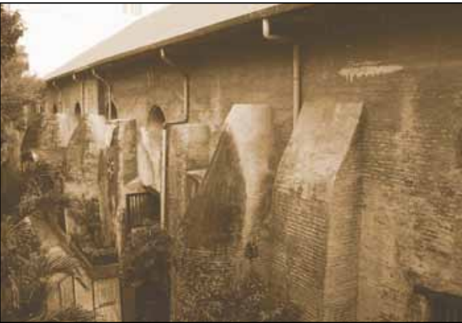
North wall of the church, with its numerous buttresses
