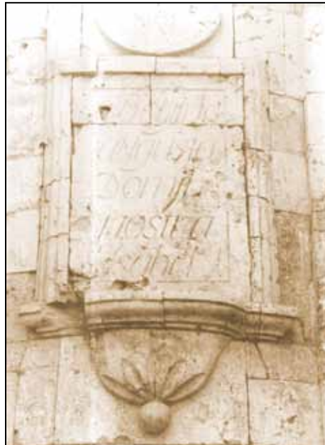
Rightmost panel of the façade referring to Narciso Claveria, governor general from 1844 to 1849. This indicates that a major part of the façade was concluded in the late 1840s, during the tenure of Fr. Yus.
