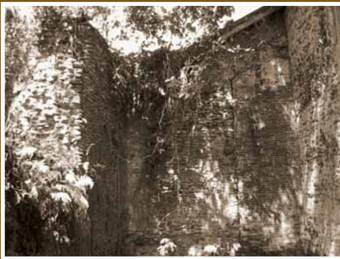
The flanks of the narrower new apse as it met the old transept were closed in with brick. This is the view inside the space between the wall of the old north transept (to the left) and the new apse to the right.
