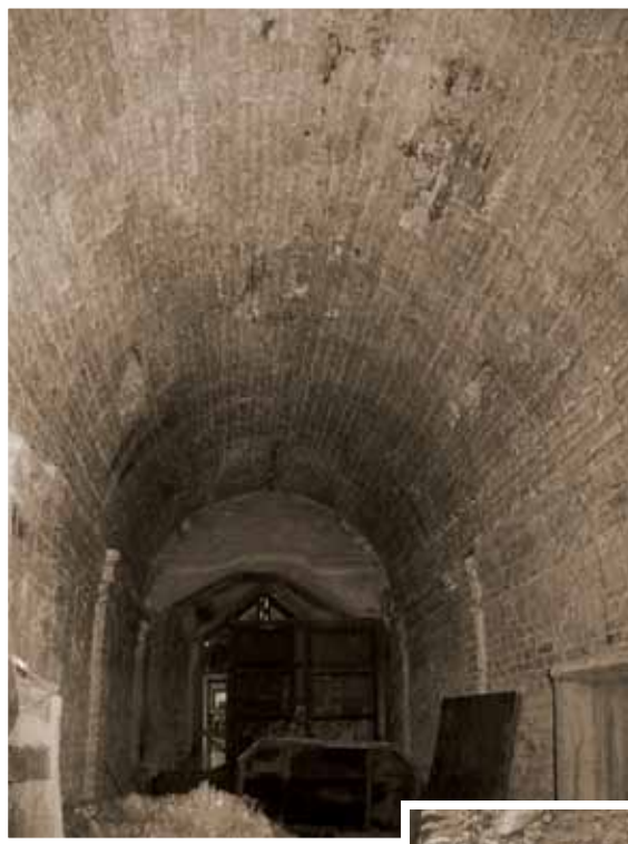
Barrel vault inside the bodega, built of finely fitted brick.
