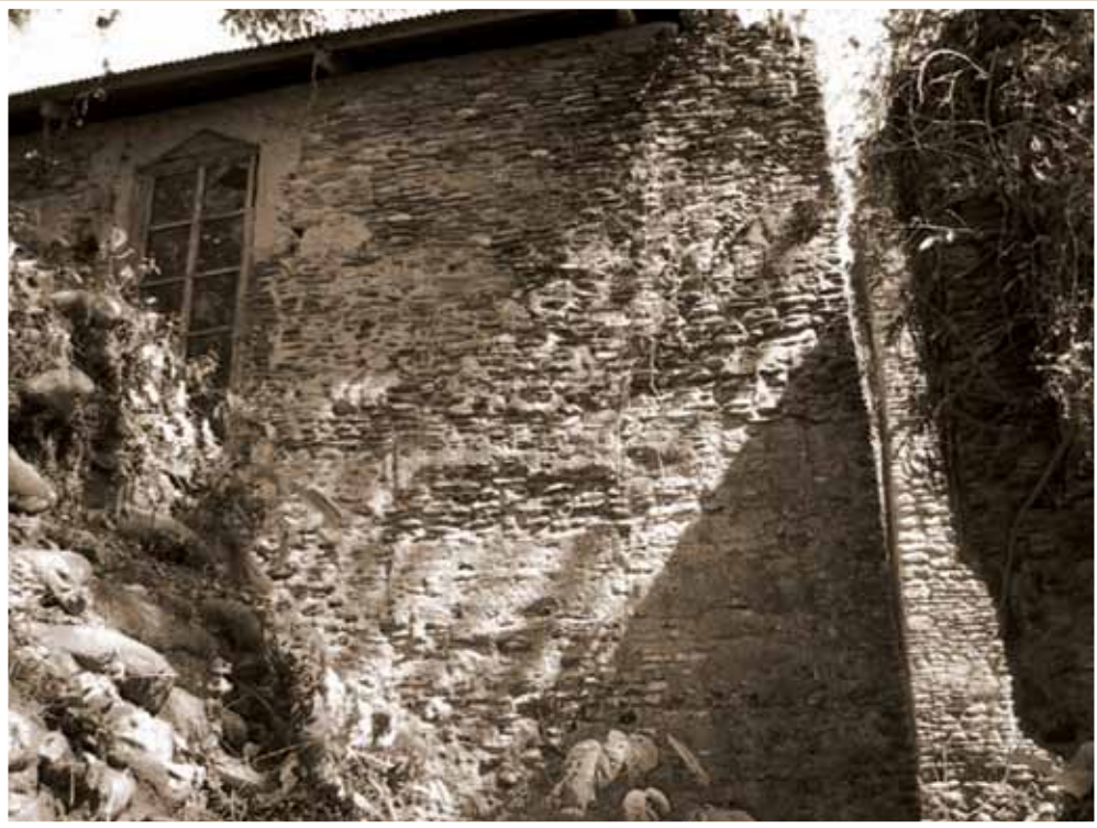
The northern end of the new apse. A crevice of light marks the narrowness between the new and old sections.
